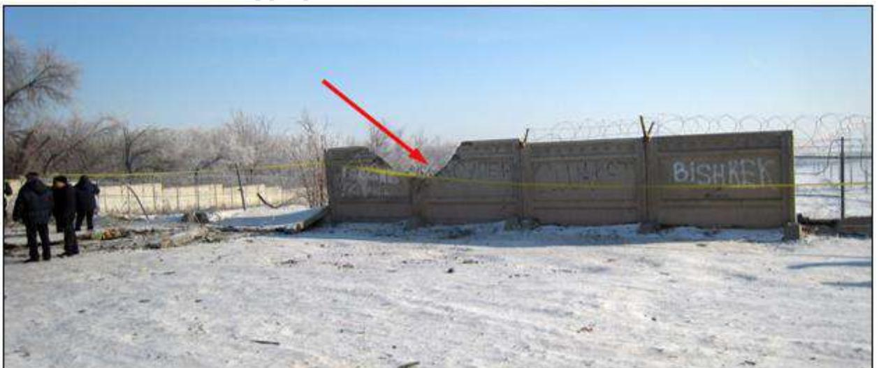
**Figure 28. Trace of LH wing engine impact with aerodrome barriers (indicated by arrow),
